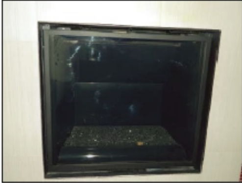
Figure 98: Frame secured to the Unit
