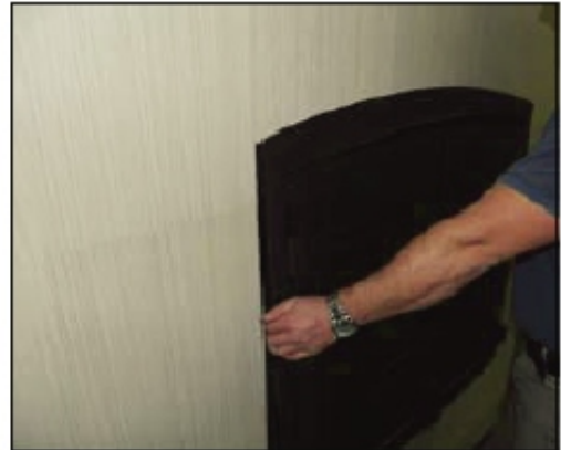
Safety screen installed
