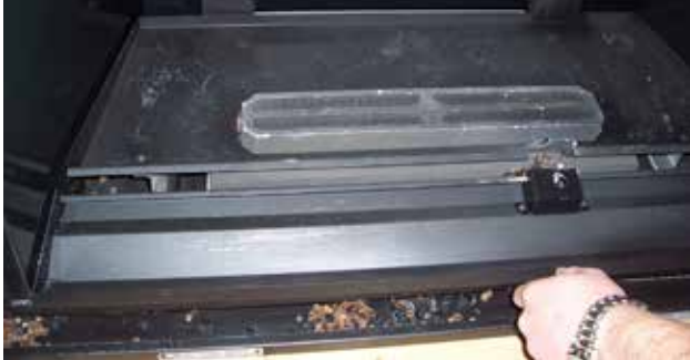
Figure 63: Lift Out Front Panel
