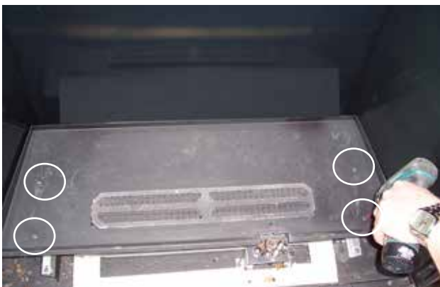
Figure 64: Burner Screw Locations
