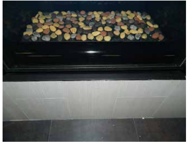
Figure 102: Completed Trim install
