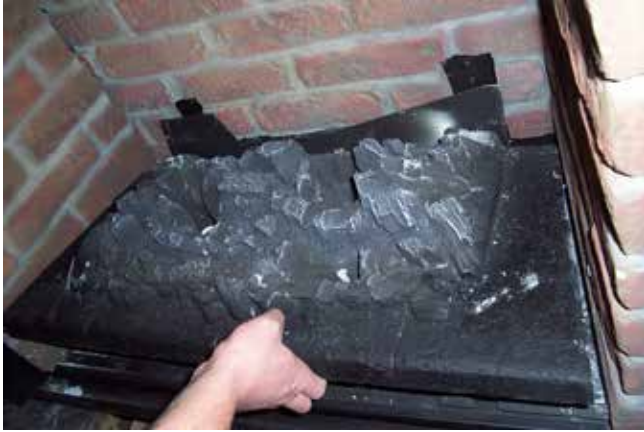
Figure 79: Burner Removal
