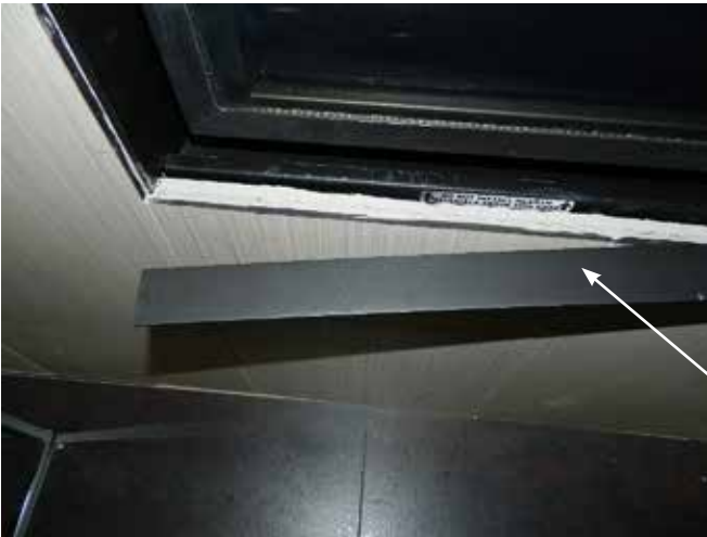
Figure 101: Top View - Sliding trim into place
