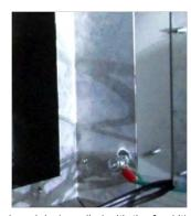
10. The fan control module (supplied with the fan kit) secures to the side access panel. Remove 2 top screws and loosen 2 bottom screws to remove the side access pane
