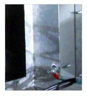
16. The fan control module (supplied with the fan kit) secures to the side access panel. Remove top screw and loosen 2 bottom screws to remove the side access pane
