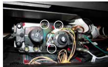
Remove NG Stepper motor and replace with LP Stepper motor
