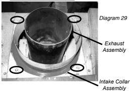
12) From the outside rear of the firebox, install the intake cover plate with 4 - 1/4" x 1/2" screws. Ensure all screws are tight, but do not over tighten. All 4 screws must be used.
