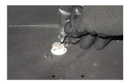
14) Install two light diffusers on to the base tray.
