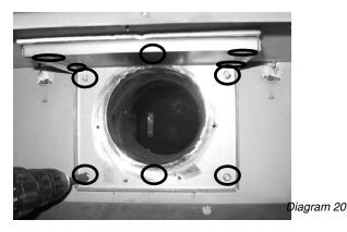
4) From the outside rear of the firebox, remove the intake collar assembly. Remove the 4 - 1/4" x 1/2" screws.
