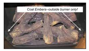
12. Test fire to ensure proper light off (make sure flame flows smoothly from one end of burner to the other. If there is any flame hesitation, check that area for any blockage of the burner port.
