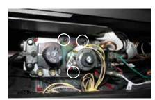
Pull off the pilot cap to expose the pilot orifice.
