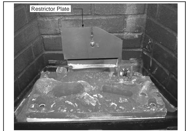
Figure 9 - Loosen screw to adjust restrictor plate.
