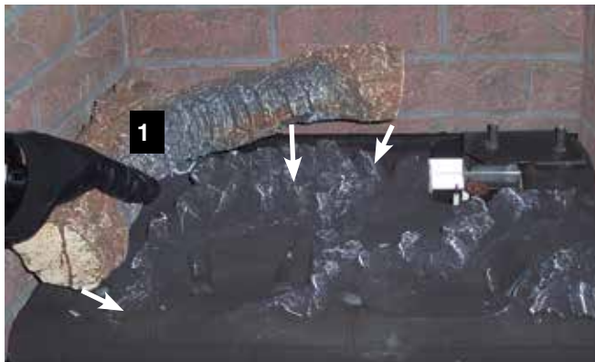
Log 1 location on burner
