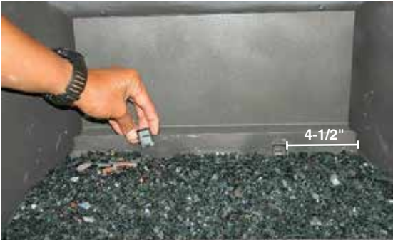
Log bracket install
