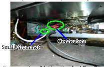
Attach the connectors (black and red) of Fan Grey wire to the IFC connectors (black and red).
