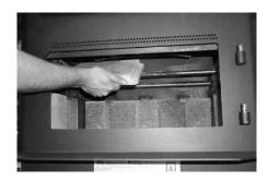
Tilt the first Baffle Brick down and then slide the 2nd Baffle Brick up and back. Reposition both baffle bricks flat on the air tubes.
